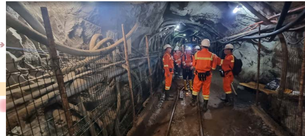
H 2 drainage boreholes at L17
